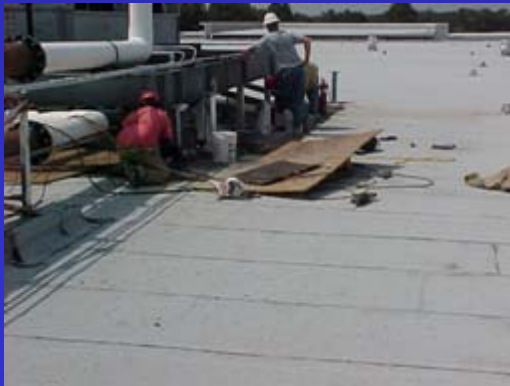
Energy efficient light colored roof at the new Sheriff's central Operations Center
